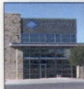
Swift-Train's San Antonio facility.
